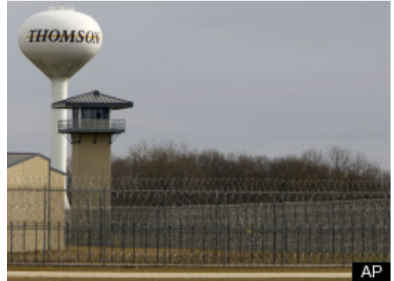
Stuck in Thomson Prison. The federal government went around Congress to buy the empty prison with no plan to fill it. Now the taxpayer is footing the $2 million maintenance bill.
